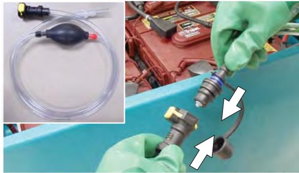
4. Submerge the other end of the hand pump hose into a bottle of distilled water
